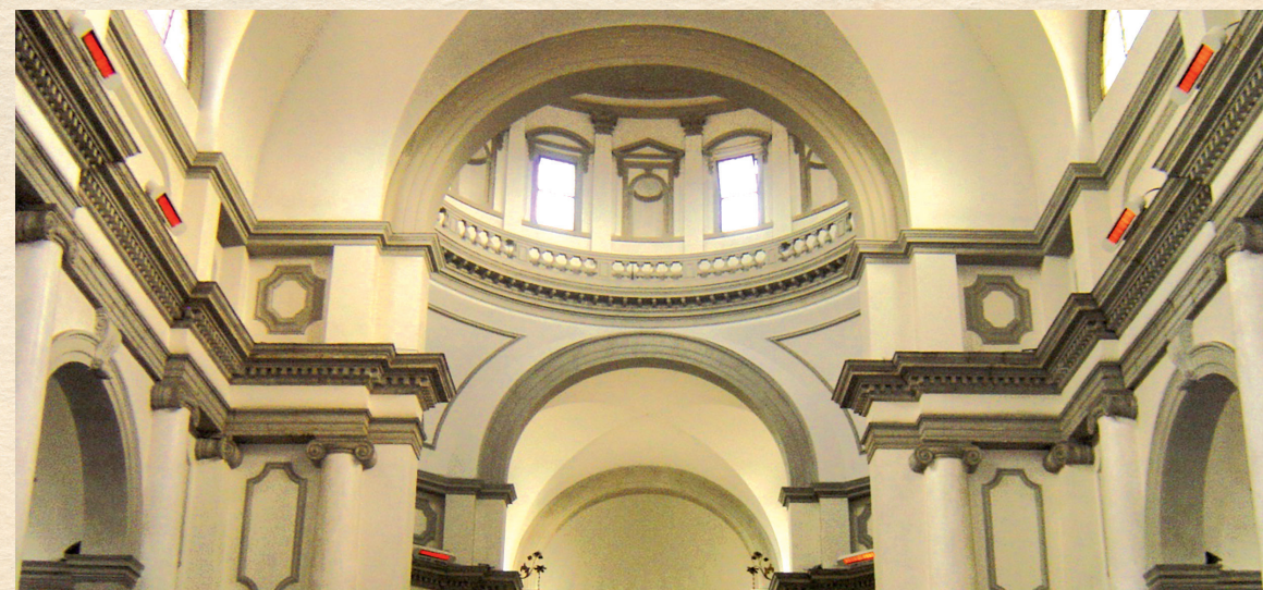
SUNRAD radiant heating system in the Cathedral of Castelfranco Veneto - Treviso - Italy
